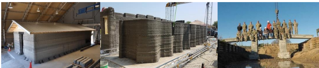
Figure 1.8. 3DPC Structures Built as Part of the ACES Project Carried Out by the US Army Corps of Engineers [24]
