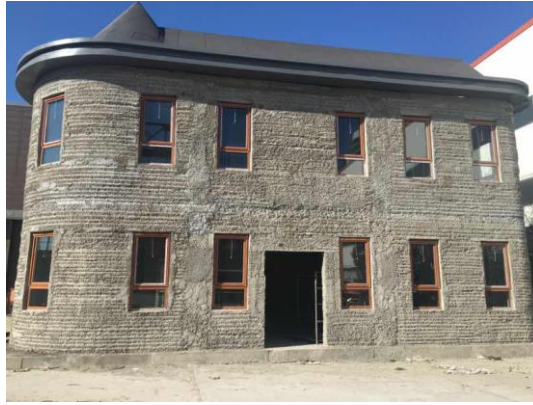
Figure 1.7. The Building Printed by the Winsun Company [23]
