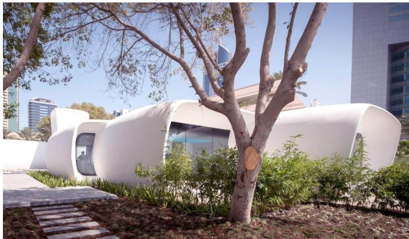
Figure 1.4. Office of the Future- 3D Printed Office; a Fully Functional Building with Electricity, Water, Telecommunications and Even Air Conditioning Systems [17]
