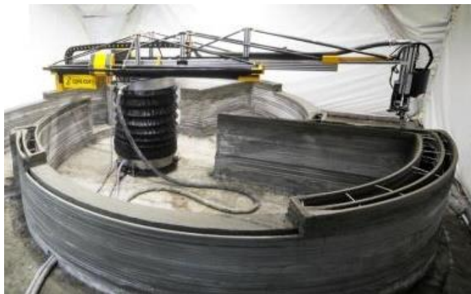
Figure 1.6. The Entire Construction Cost was Around $10,000 and it can Withstand Temperatures as low as -35^{\circ}\text{C} . This Type of Technology can Provide an Alternative to Traditional Construction Methods, Thereby Creating Affordable Housing [21]
